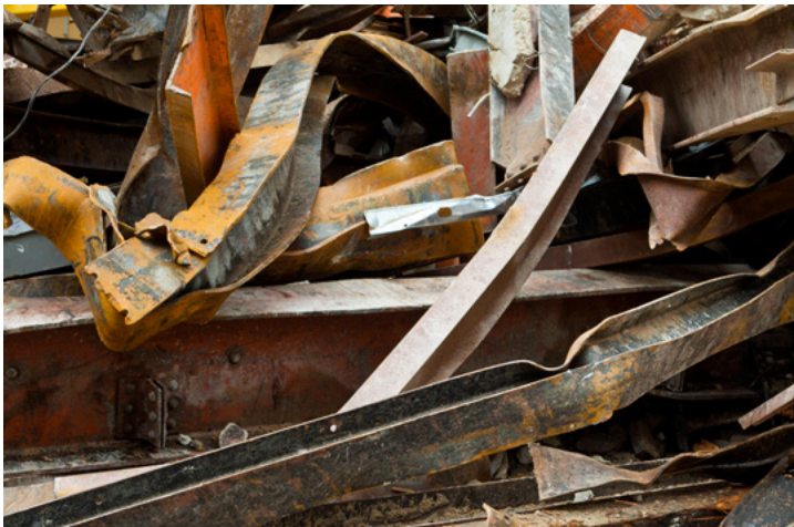
Debris from the demolition of an unidentified building.
