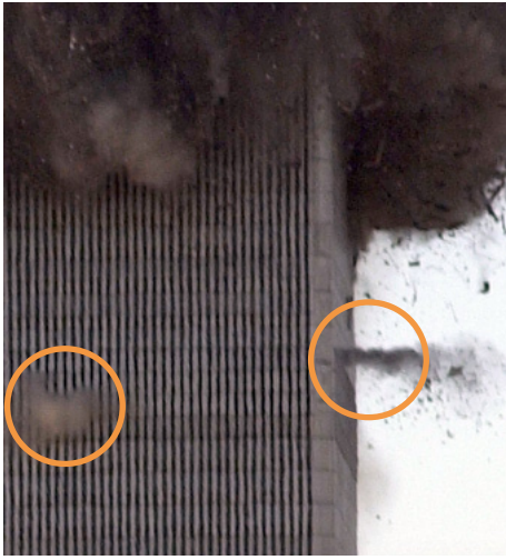
High-velocity bursts of debris, or “squibs,” were ejected from point-like sources in WTC 1 and WTC 2, as many as 20 to 30 stories below the collapse front.
