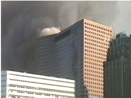
This video, which surfaced in 2008, clearly shows vertical sequences of explosions and window breakage as WTC 7 begins to collapse. It can be viewed at http://AE911Truth.org/downloads/video/WTC7-West.mp4
