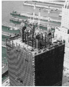
WTC 1 during construction.
