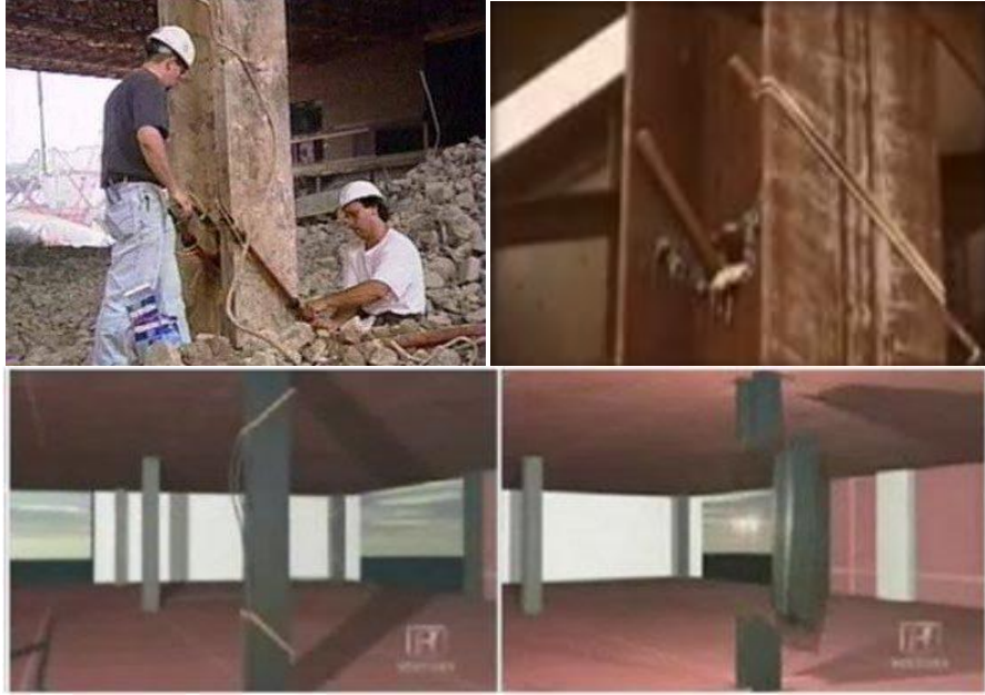
Figure 1: Examples of Demolition Explosives Placed at Angles
