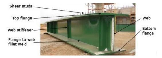
Shear studs, as seen in the two diagrams, are short unthreaded bolts welded to the top flange of a steel girder. The shear studs become embedded in the above concrete flooring slab to form a composite beam, which then acts structurally as one beam which is stronger than the steel beam.
