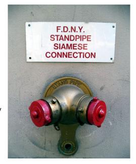
In the unlikely event that water was limited to the building from both separate mains water supplies being broken, or simply in order to boost the system, the sprinkler system also had the capacity to be charged with water from external Fire Department connections to the building (siamese fittings). These were located on outside walls at Washington St., West Broadway, and the loading dock.
