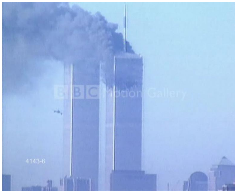
Fig. 6: UA 175 Three Seconds and Approximately 0.45 Miles Before Impact
