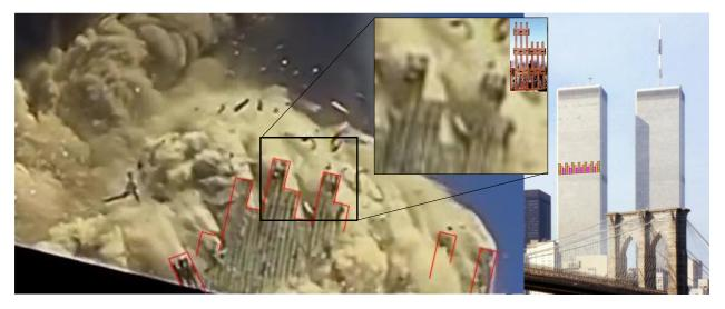
Figure 1: Eight or more contiguous perimeter column sections are seen propelled (left) from their initial location near the 80<sup>th</sup> floor (right). At this point, they have traveled over 200 feet from the South Tower wall.
