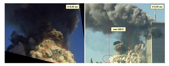
Figure 4: Location of the "surfing" columns from the southeast (left) and the northeast (right) at 6.25 second after the hinging motion begins.
