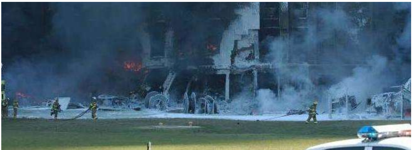
Figure F-9 Spools with fire mostly extinguished
