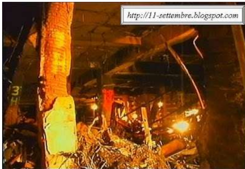
Figure G-1 Curved and abraded column
