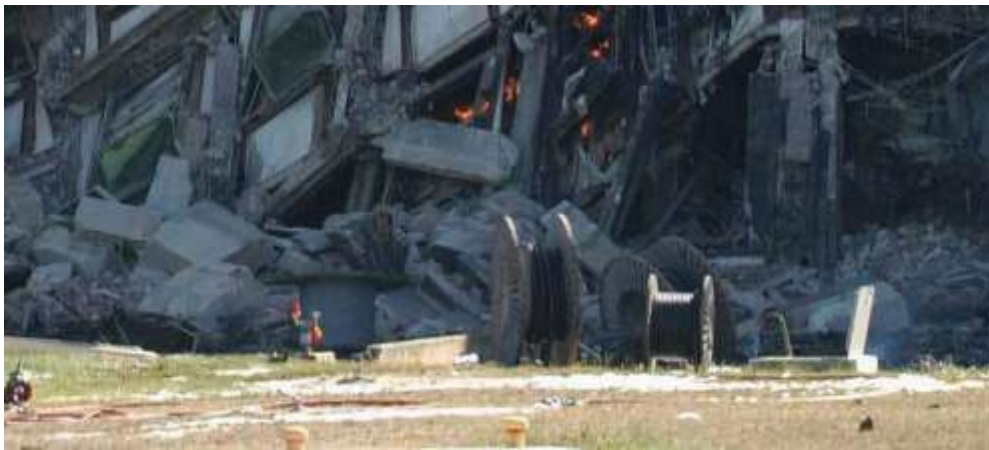
Figure F-7 Low concrete wall and small spool
