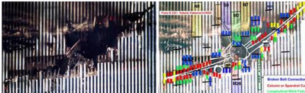
Left: WTC1 north face; Right: Damage relative to a Boeing 767. Note that only the tip of the starboard (right) wing cut through the 98th floor.
