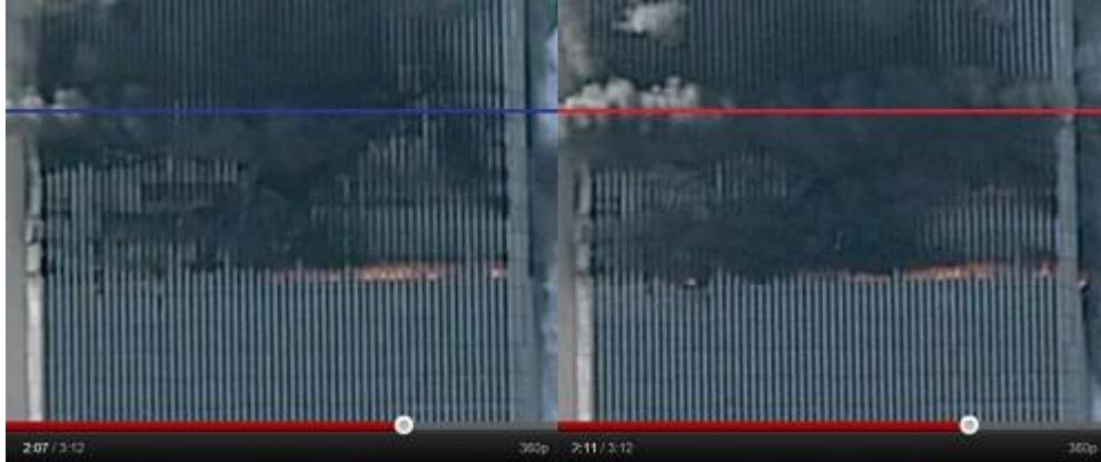
Left: WTC1 before collapse; Right: WTC1 at start of collapse. Blue line denotes 98th floor. Red line denotes approximate area of collapse initiation. Stills taken from video of North Tower collapse: https://www.youtube.com/watch?v=xGAofwKAOLo
