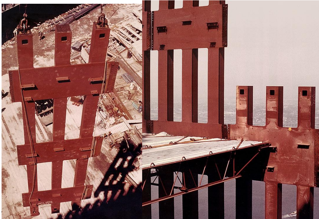
Figure 2. Perimeter columns in WTC towers. From NIST.
